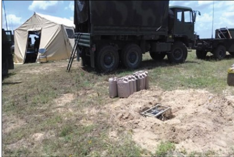
Figure 10-5. Diminish noise by placing generators in hand-dug holes.
