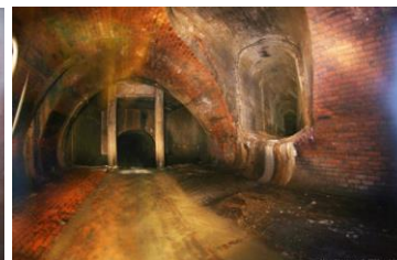
2B: Civil works (Sewers, Subways, & Aqueducts)
