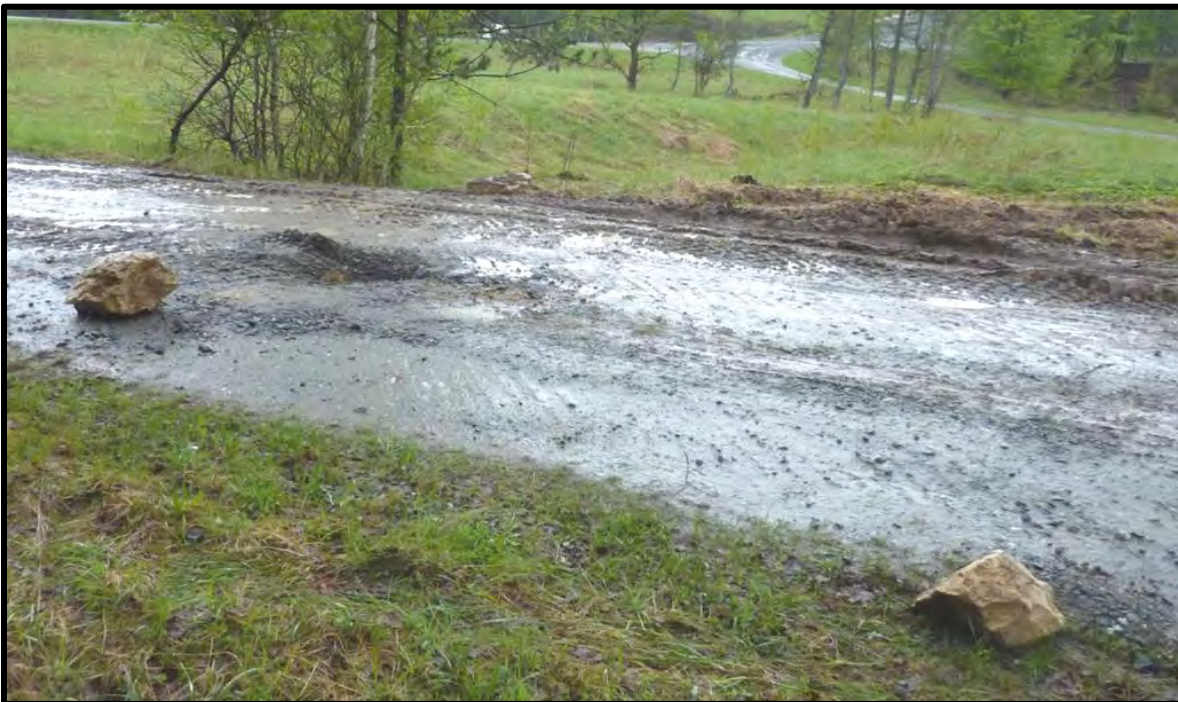
Figure 2-22 Rocks Placed to Channelize Vehicle Traffic
