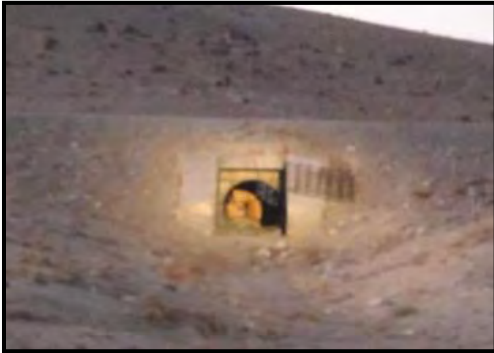
Figure 3-30 Danger Area- Culvert with IED Inside
