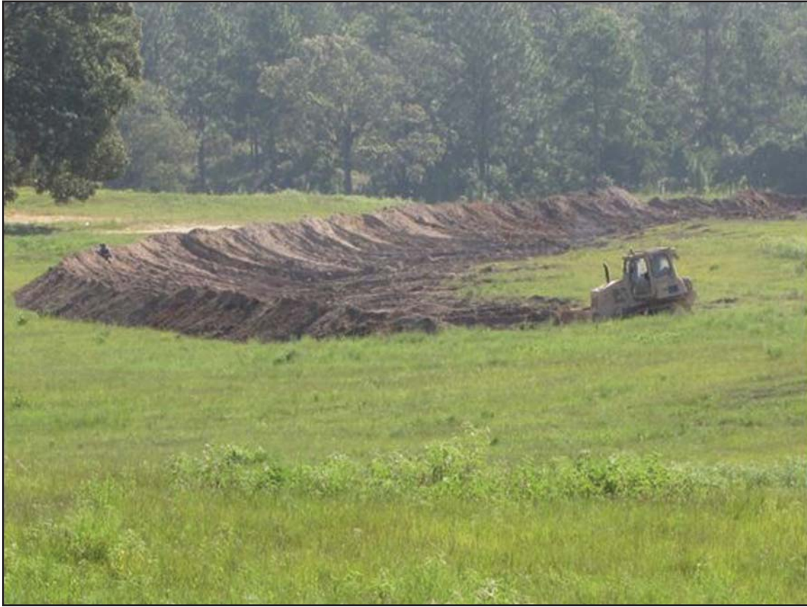
Figure 10-1. Carving the berms for the field artillery.
