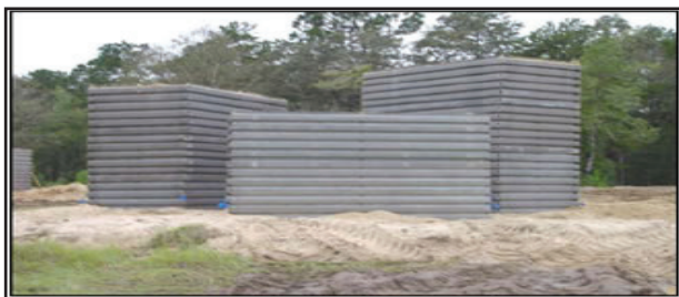
Figure 3-15. Metal Container Barrier
