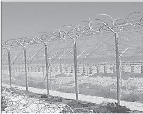
Figure 3-28. Chain-Link Fence with Razor Wire and Barbed-wire Outriggers
