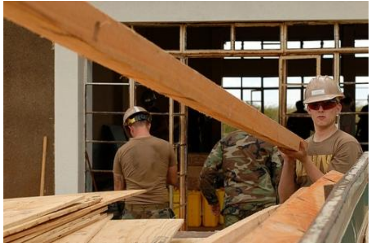
Figure 24 - Missions also include construction and rebuilding of infrastructure
