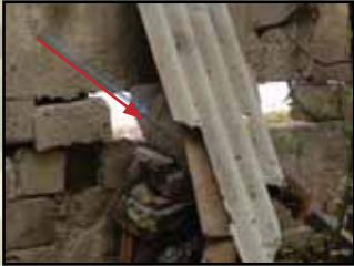
Elevated IED Concealed Behind Wall - Somalia
