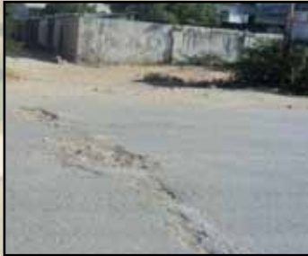
IED Buried in Pothole - Somalia
