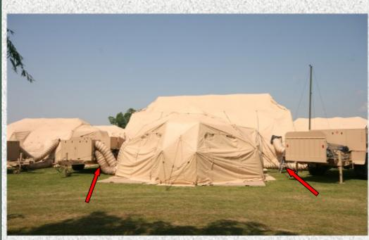
On the right hand side of the picture, on the low return duct, it is straight. This allows maximum air flow throughout the duct.
