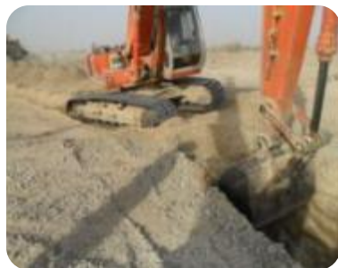
Using Material Handling Equipment (MHE) to clear and expand irrigation canals
