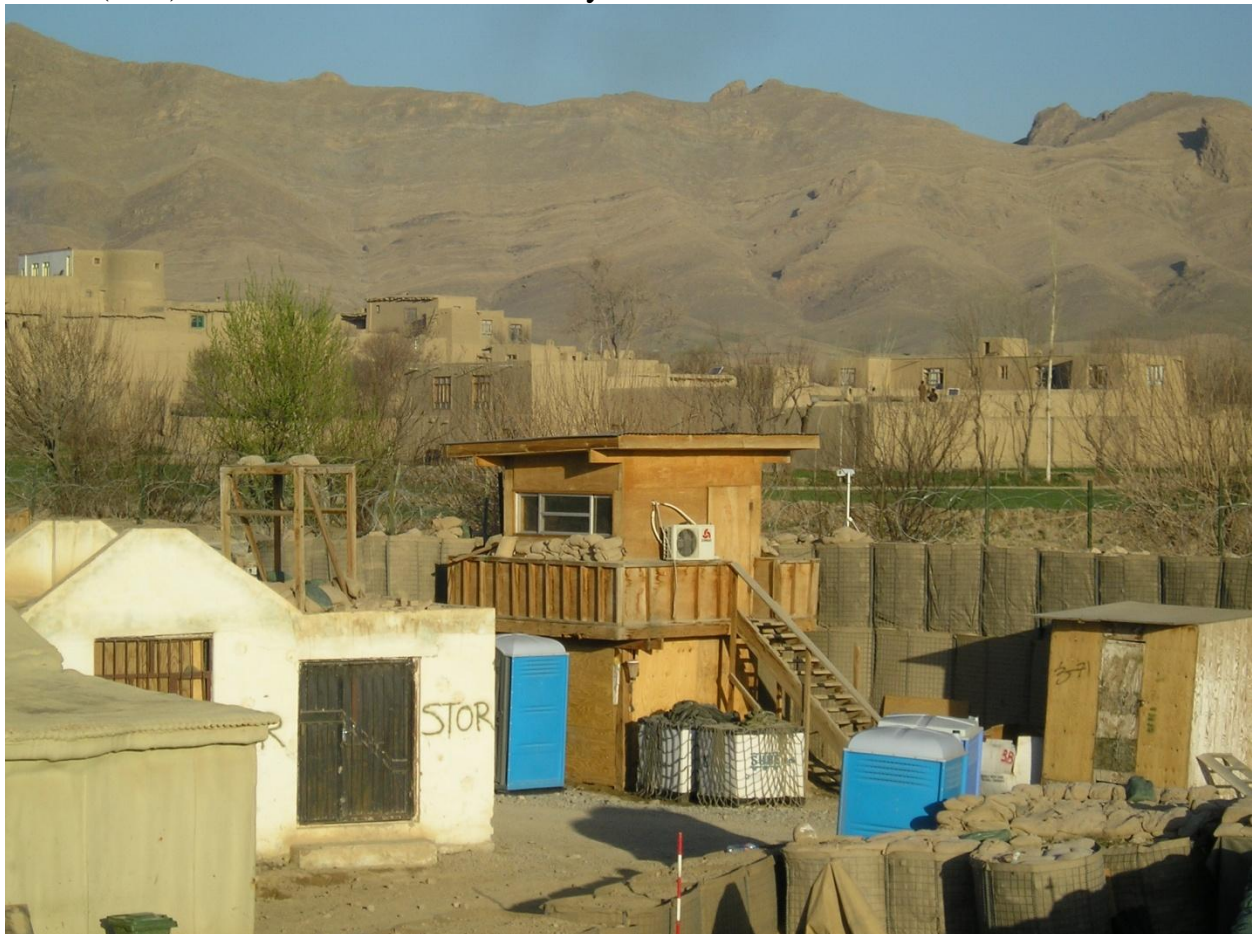
Figure 2 Guard tower at BBK with HESCO Barriers.
