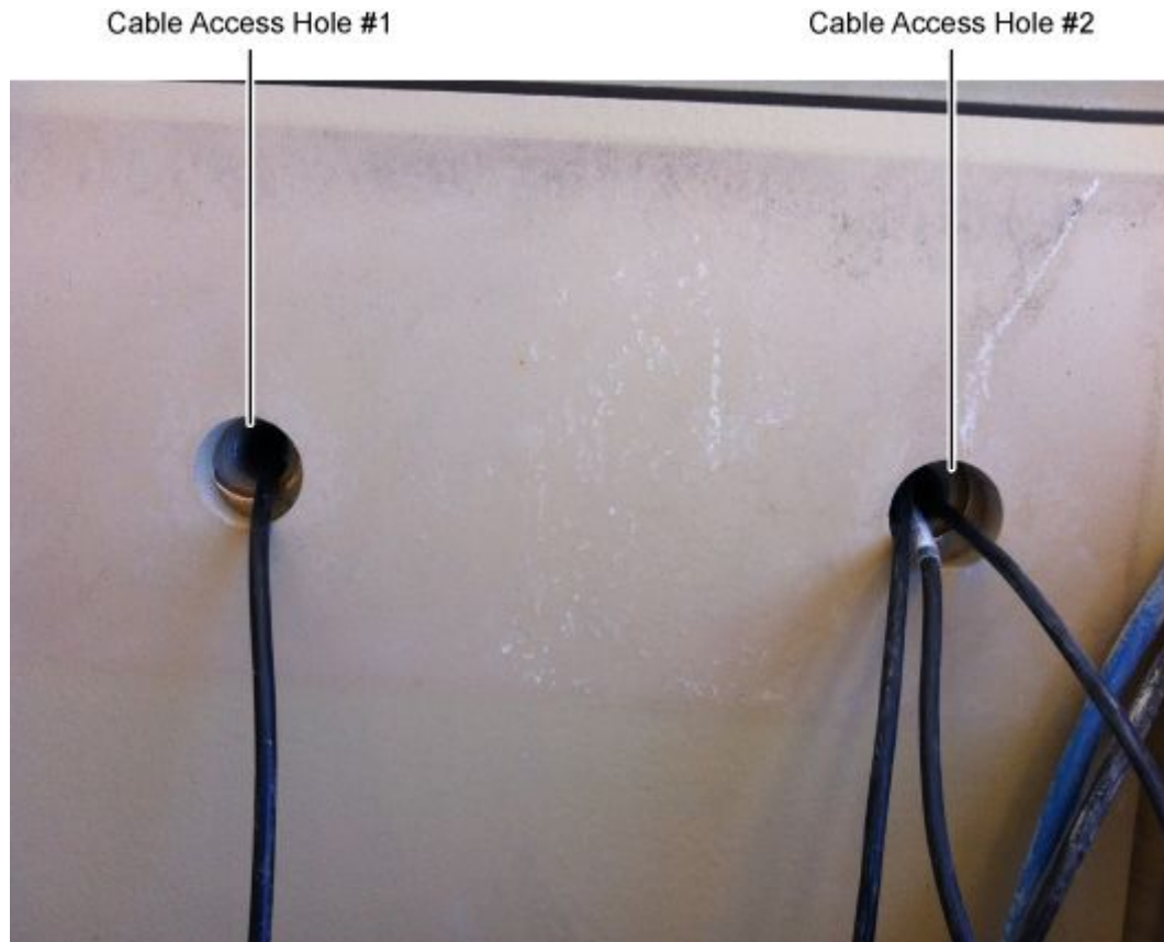
Figure 4-30. Cable Access Holes Behind Gunner's Position (Outside View)
