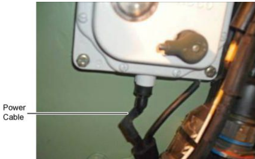
Figure 4-49. Dome Light Power Cable
