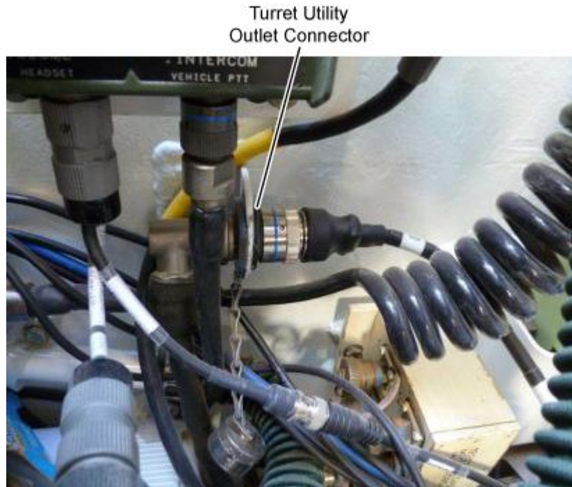
Figure 4-13. M1A2 Power Cable Connected to Utility Outlet Connector
