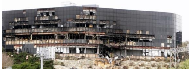
Damage caused when Andrew Stack flew his single-engine plane into a building housing an IRS office in Austin, TX.
