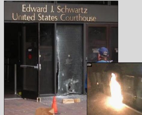
U.S. Courthouse in San Diego, CA
